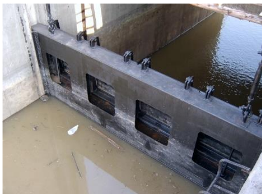
Figure 3 Hinged Flap Gate
