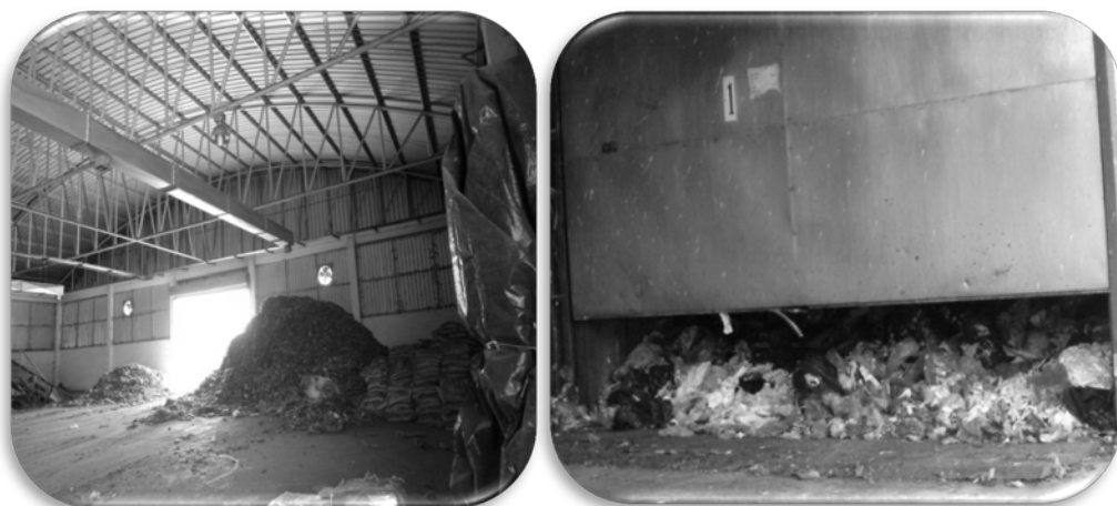
Figure 1 Show untidy collecting of waste in the plant
