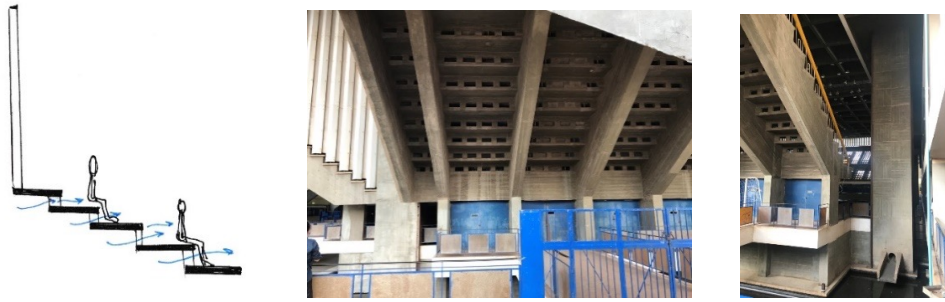
Figure 5 Hole punches underneath of the audience seats provide a soft lighting and ventilation into the indoor arena. Photo by Ty Pisith, March 8, 2018.
