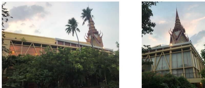
Figure 16 Photos showing from the south elevation foyers with openable linear windows, that can be used as air ventilation access into the building. Photo by Ty Pisith, March 8, 2018.
