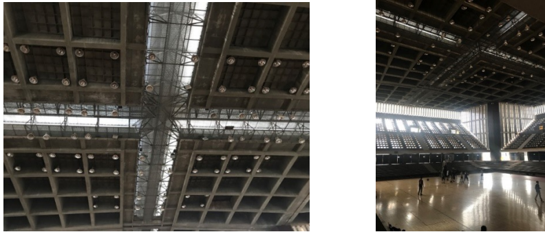
Figure 8 The opening space in between the four main rooftop structures is covered by an opening gable roof that allow indirect sunlight and air circulation inside indoor arena. Photo by Ty Pisith, March 8, 2018.
