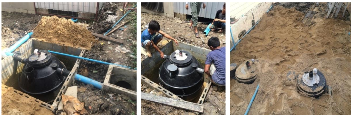
Figure 2 Four units of integrated CST and UF system (in the stage of the school construction)
