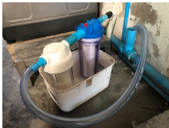
Figure 1 Installation of a two-stage filter system
