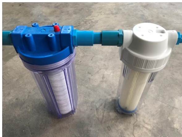
Figure 1 Installation of a two-stage filter system
